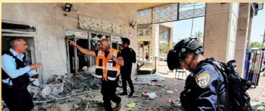
Damaged building in southern Israel by Hamas rocket fire
