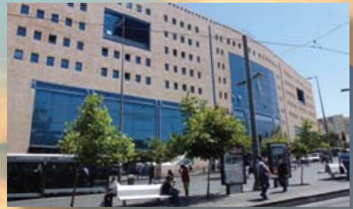
CFI's rented facilities
